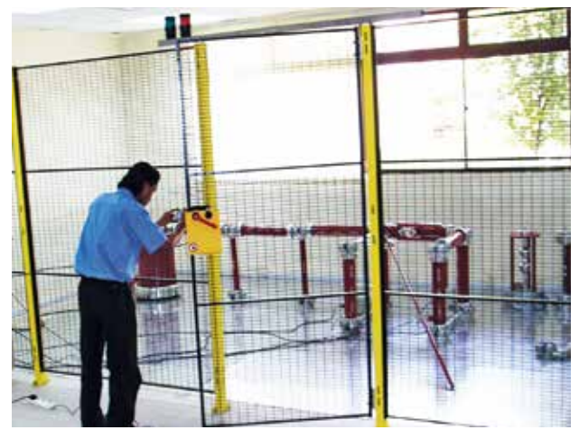
Installation of Safety Fence
